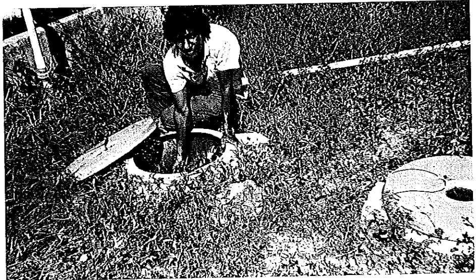
Cromaglass Batch Treat System serves several hotel resort cottages.
