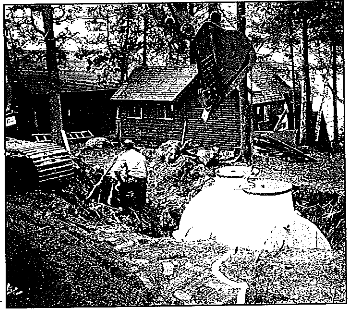
Treatment System being Installed on Moosehead Lake shoreline.
