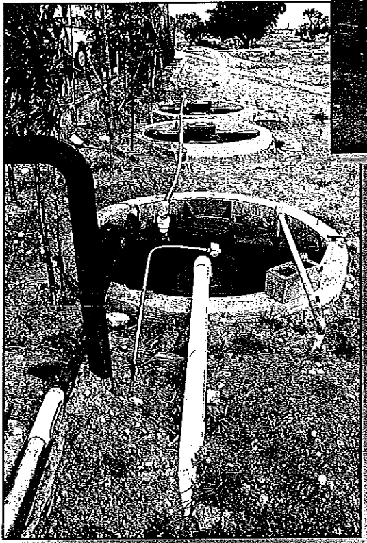
Treated Effluent Holding Tanks
