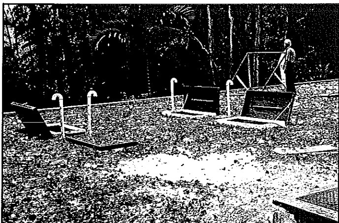
The hotel of Villa Nova is served by Cromaglass Model CA-150 (15,000gpd) wastewater treatment system. Treated effluent
